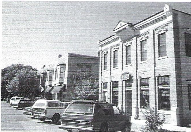
A new mixed use storefront building fits into the main street
